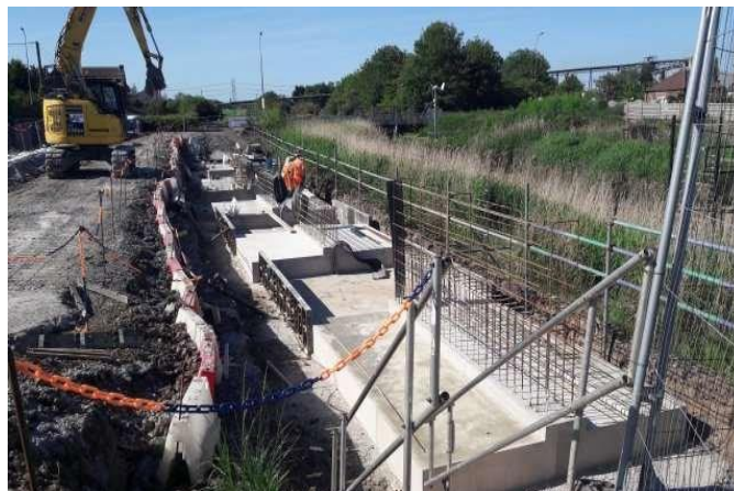
Flood wall foundations being cast along East Drain
