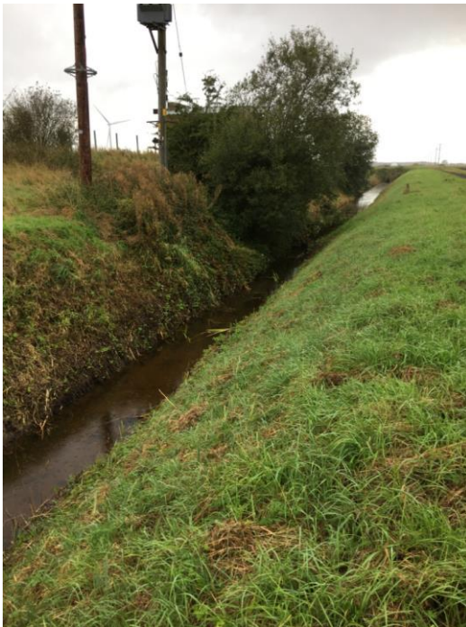
Cross Drain toward pump station
