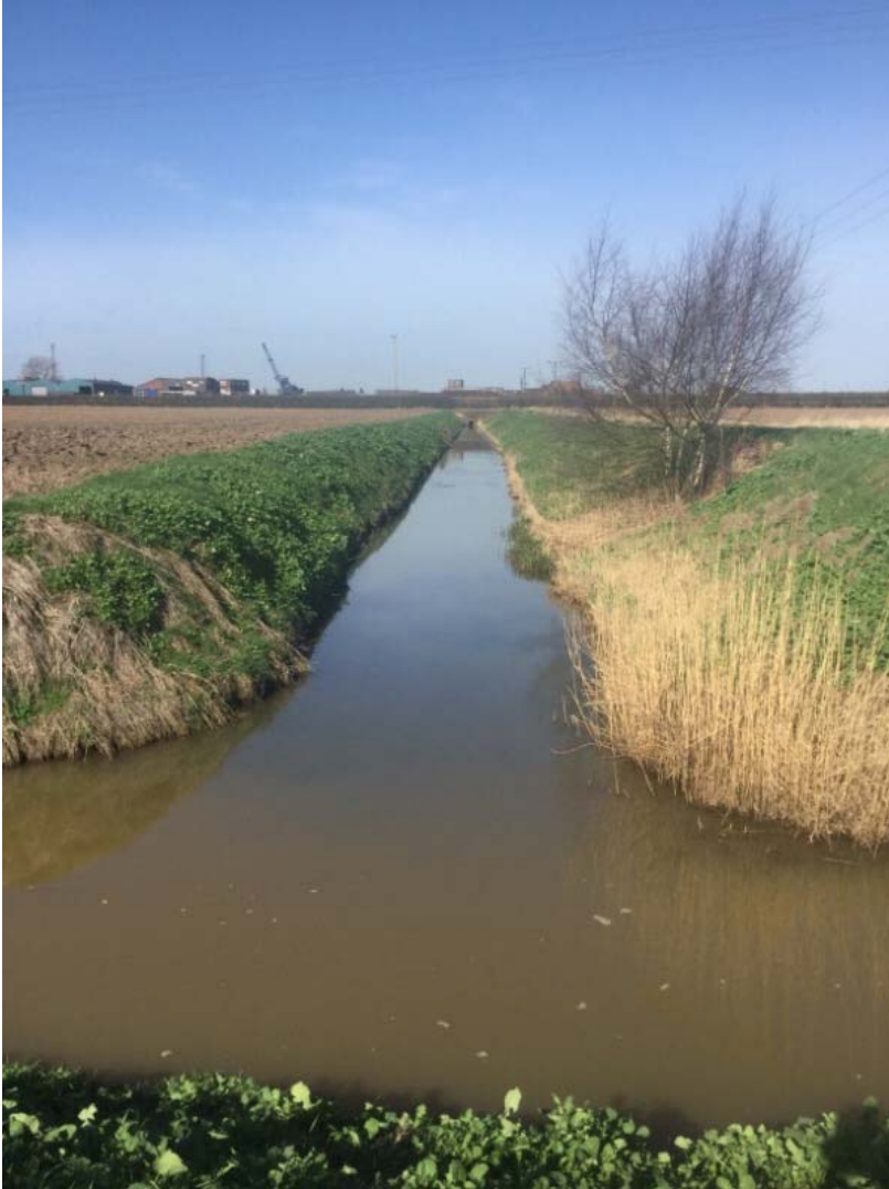
Junction with Neap House Drain
