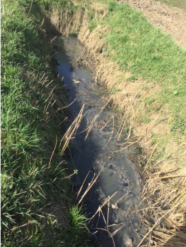
Neap House Drain pollutant
