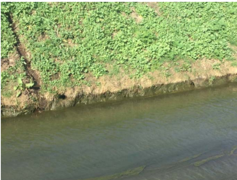
Carr Dyke Road Drain North, numerous burrows, large differential in water levels from pumping, not necessarily conducive to optimum water vole habitat. No evidence of environmental best practice.
